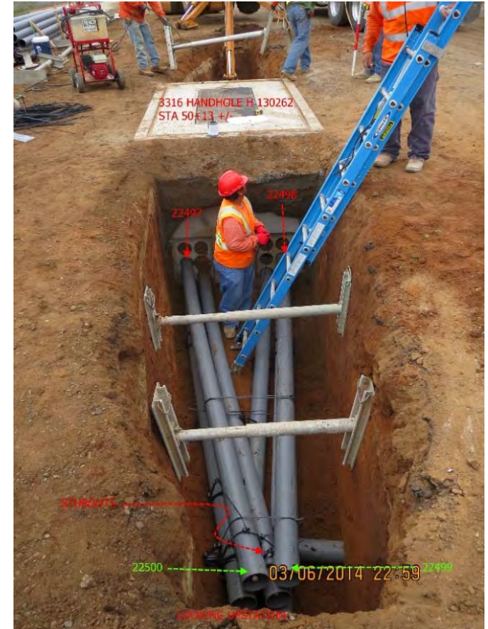
B. Typical 12-kV Duct Bank
