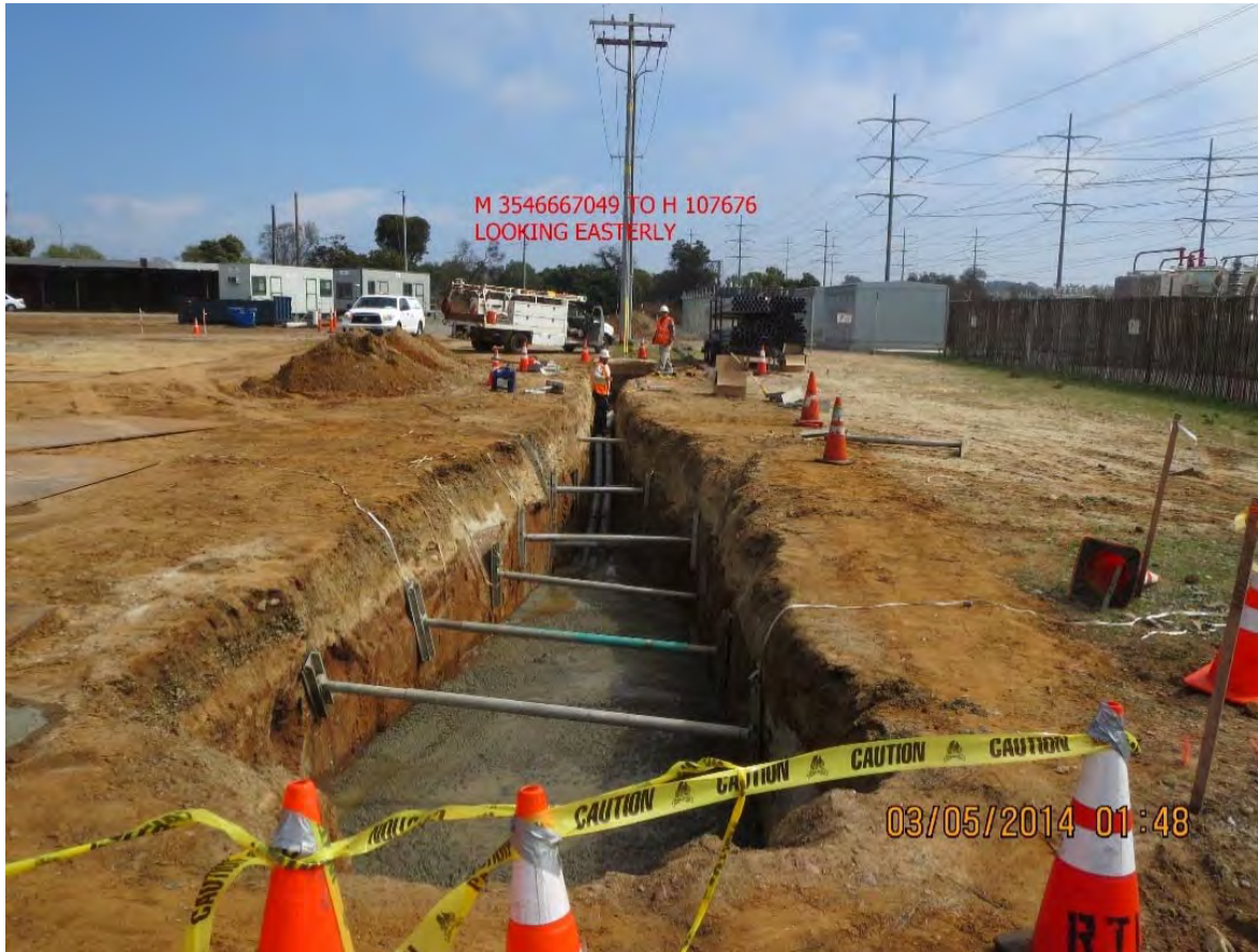
A. Typical 12-kV Trench
